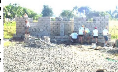
The New Restrooms For The School
